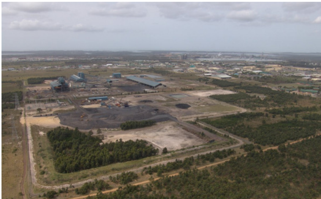
Figure 3: Photographs showing development status before and after industrial development; (Estuary in 1970, view south west from the coast) 3 and (Grassland in 2009, view south from inland) 4 .
