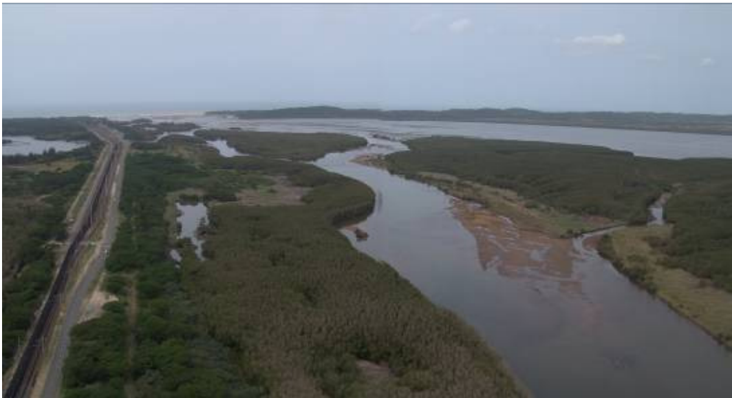
Figure 4: Dyke with railway and road separating the harbour (left) from the estuary (right).
