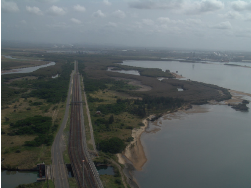
Figure 4: Photograph of the berm that was constructed to separate the harbour (on the right) and the estuary (on the left)
