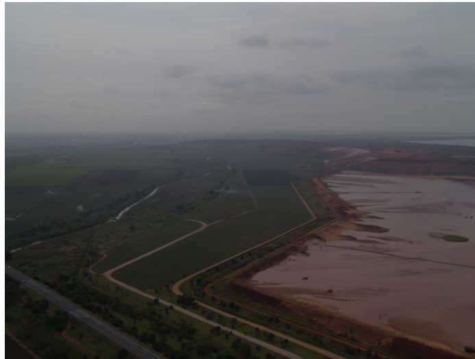
Figure 31: Slimes dam to support the Hillendale Mining Operations (Photo: D van Vuuren)
